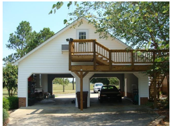
Rear of garage
